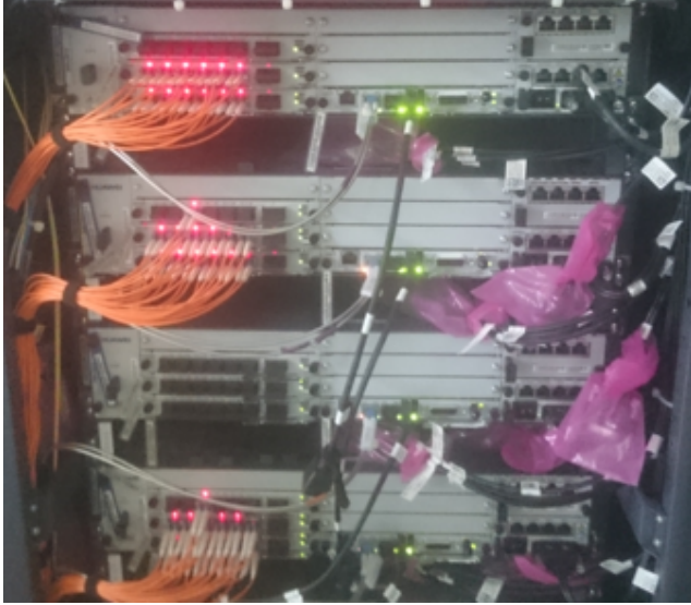
Fig. 5: BBU pool used in central location of C-RAN in Cekmekoy district of Istanbul.
